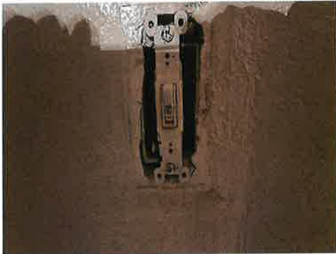
1218-1 Plaster Typical Interior Walls/Ceilings
