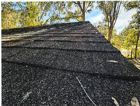
1218-3 Asphalt Shingle/Tar Typical Exterior Roof
